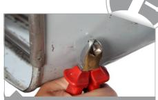
There are 2 options for riveting either with a snap die and hammer or the simpler versior with the SIP riveting pliers. 2 helping hands are helpful for the mounting. Transfix the rivets and clip off the overhang up to 3mm.
